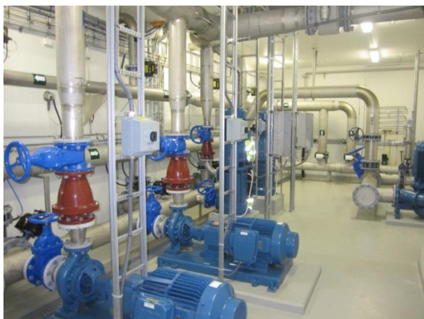
Figur 5 Rentvannspumper
